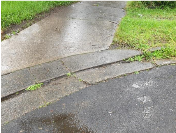
Photo 2.1-85 Cracking observed in layback to No. 24 (facing north)
