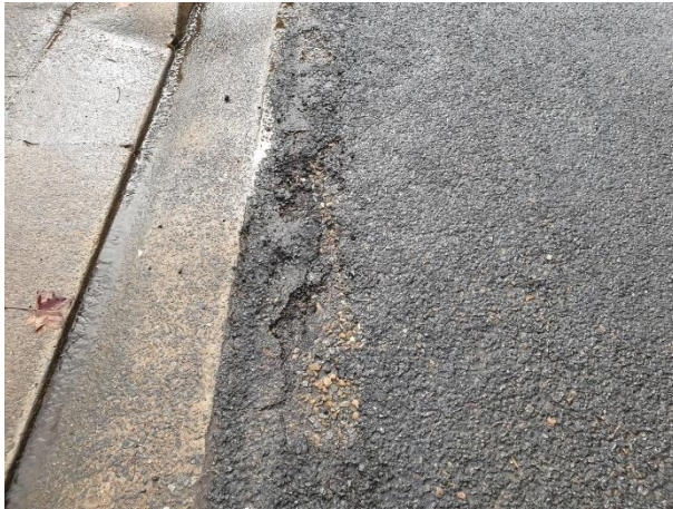
Photo 2.1-7 Deteriorated road surface adjacent driveway to No. 21
