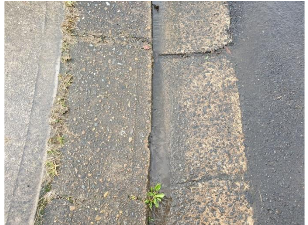
Photo 2.1-80 Cracking observed in layback to No. 22
