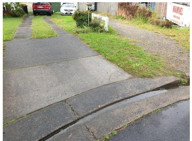
Photo 2.1-90 Cracking observed in layback to No. 26 (facing east)
