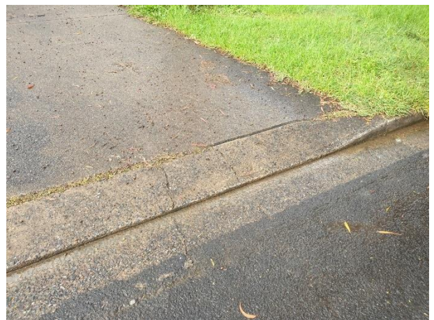
Photo 2.1-102 Cracking observed in layback to No. 30 (facing east)
