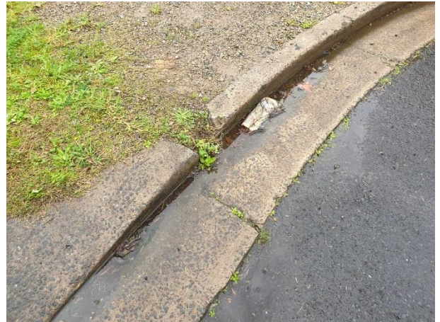
Photo 2.1-92 Chipping of kerb and gutter observed adjacent No. 26 (facing east)
