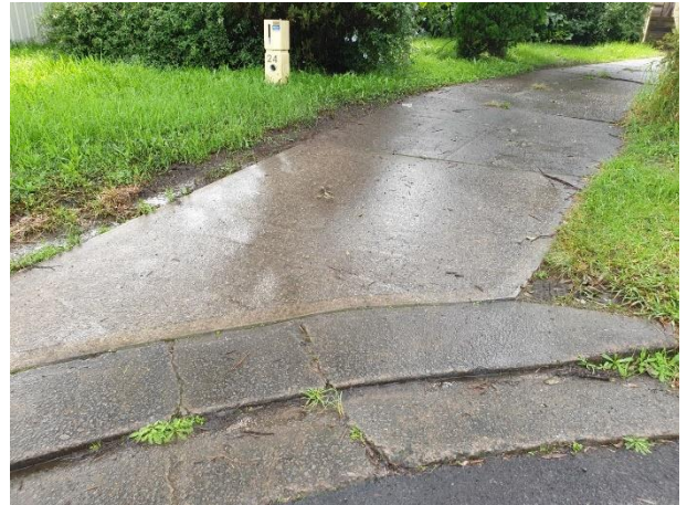
Photo 2.1-86 Cracking observed in layback to No. 24 (facing north)
