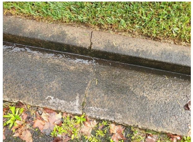
Photo 2.1-16 Cracking observed in kerb and gutter (facing west)
