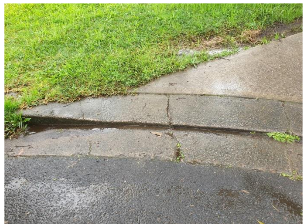
Photo 2.1-84 Cracking observed in layback to No. 24 (facing north)
