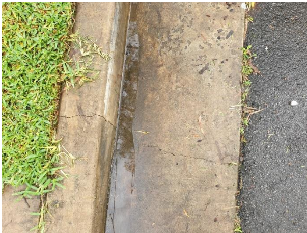
Photo 2.1-51 Cracking observed in kerb & gutter adjacent No. 13A
