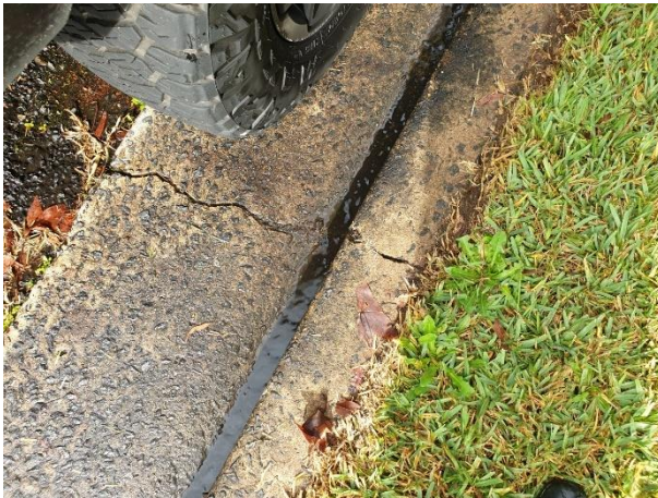
Photo 2.1-27 Cracking observed in kerb & gutter adjacent No. 17
