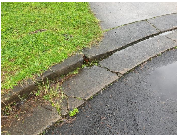
Photo 2.1-89 Cracking observed in layback to No. 26 (facing east)
