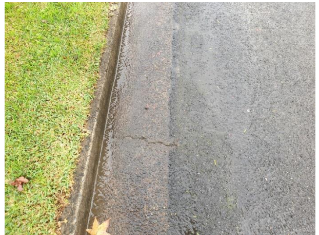
Photo 2.1-110 Cracking observed in kerb & gutter adjacent No. 32
