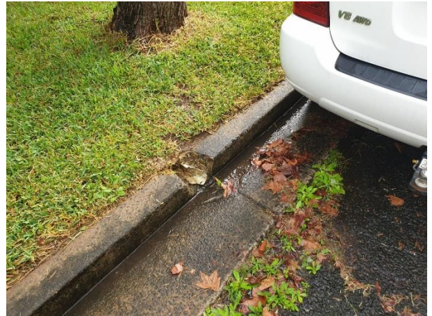
Photo 2.1-20 Damaged kerb & gutter observed adjacent No. 17 (facing north)
